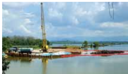
Containment of sediment for earthwork filling
