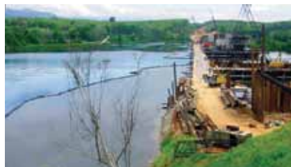
Bridge construction containment control
