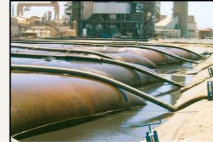
Geotube® containers at fossil fuel power plant being used to dewater fly ash.
