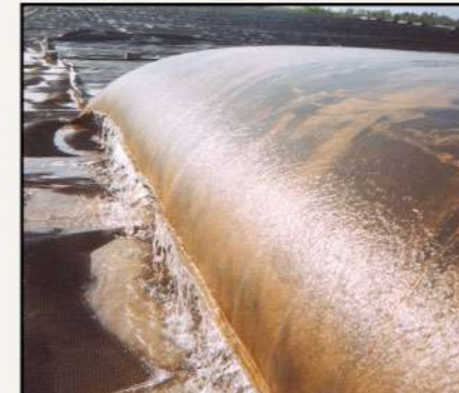
Water draining from a Geotube® container.
