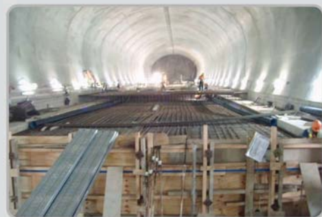
MTRC XRL 821 Shek Yam To Mei Lai Road Tunnels
