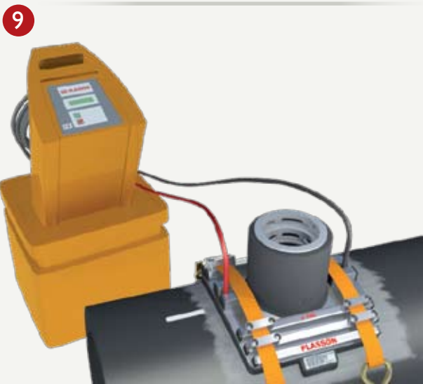
Fuse the fitting according to ElectroFusion procedures.
