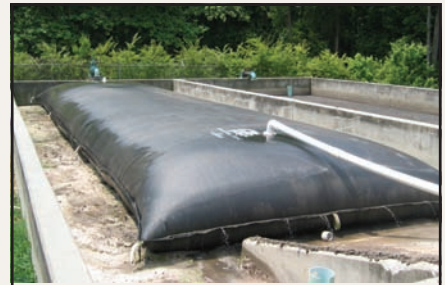
Geotube® unit in municipal wastewater treatment drying beds.
