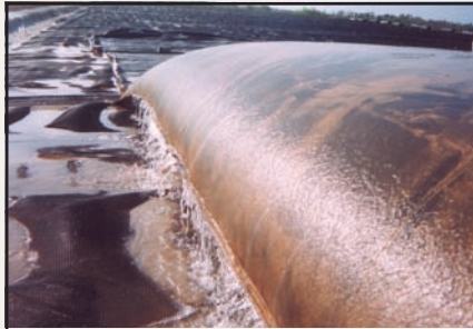
Water draining from a Geotube® container.
