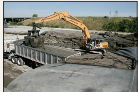
Dewatered sludge being removed from a Geotube® container with a backhoe.
