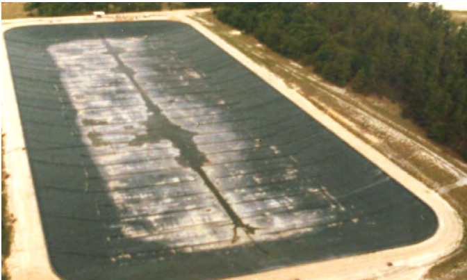
Weighted pipe cover - ideal for applications with minimal water level fluctuation
