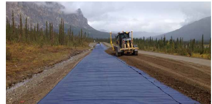
SUBGRADE STABILIZATION
