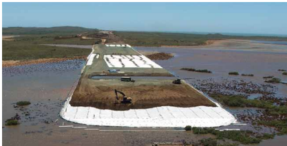
BASAL REINFORCEMENT
