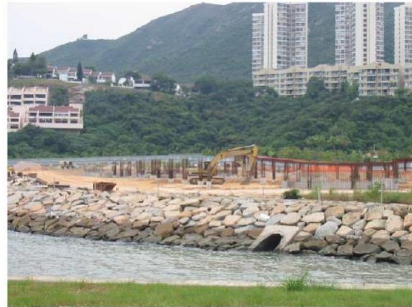
Rubble Mound Seawalls
